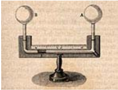
Galileo's thermoscope (Gas dilation)
